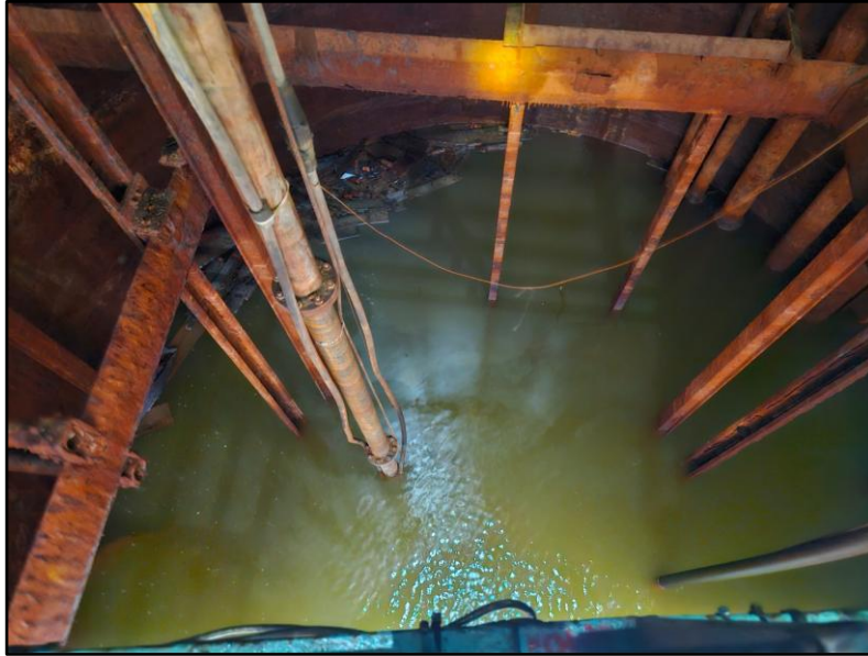
Photo 4: Mine Dewatering 500m 3 /hr (proof of concept).
