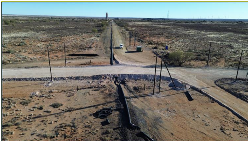
Photo 1: Dewatering Pipe and Overhead 11kV to TSF.
