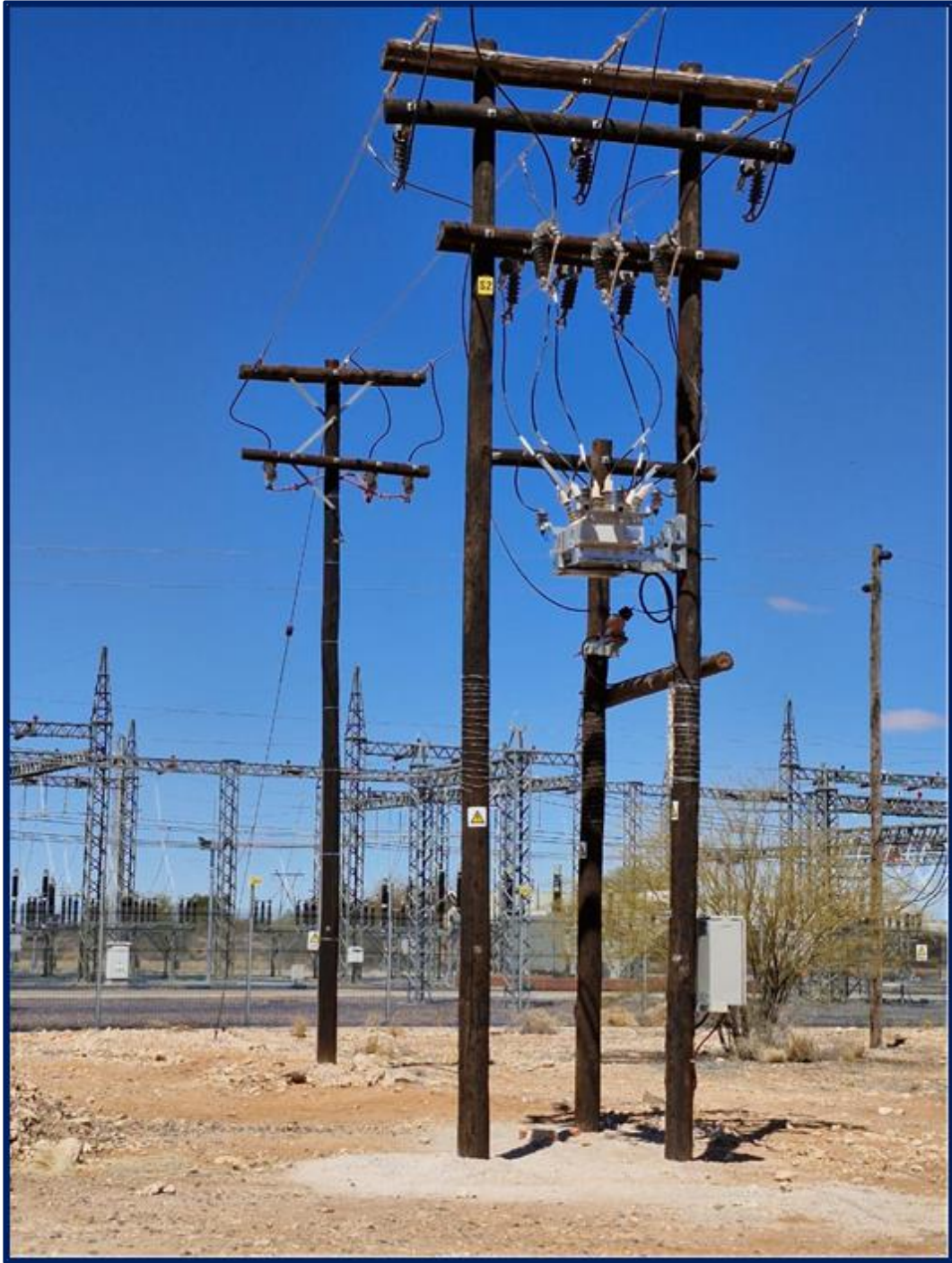
Photo 5: Cuprum Substation 15MVA tie-in to PCZM electrical reticulation.
