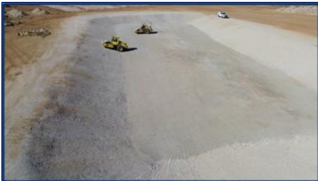
Photo 2: Construction of the 50m x 80m Overflow Sump.
