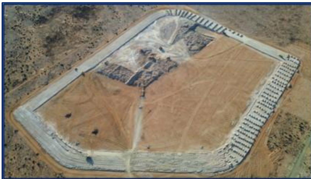
Photo 8: 13ha Storage Dam Civil Construction.
