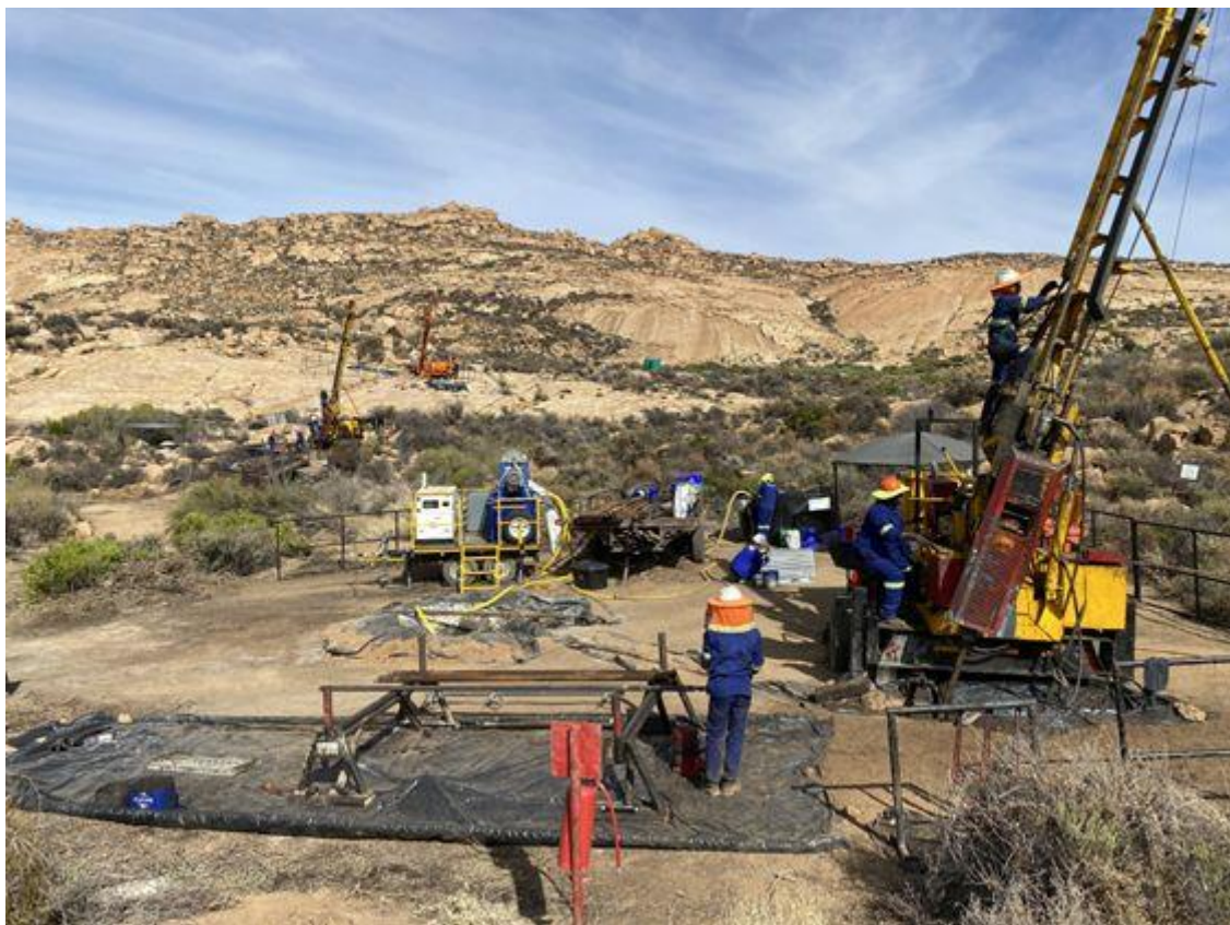
Figure 1: Drilling at FME.
