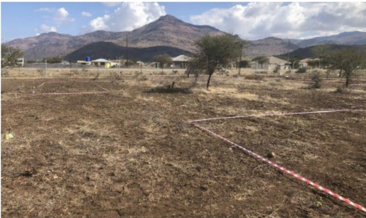
Contractor GeoMech has set out its laydown area to commence drilling within the newly-constructed security fence
