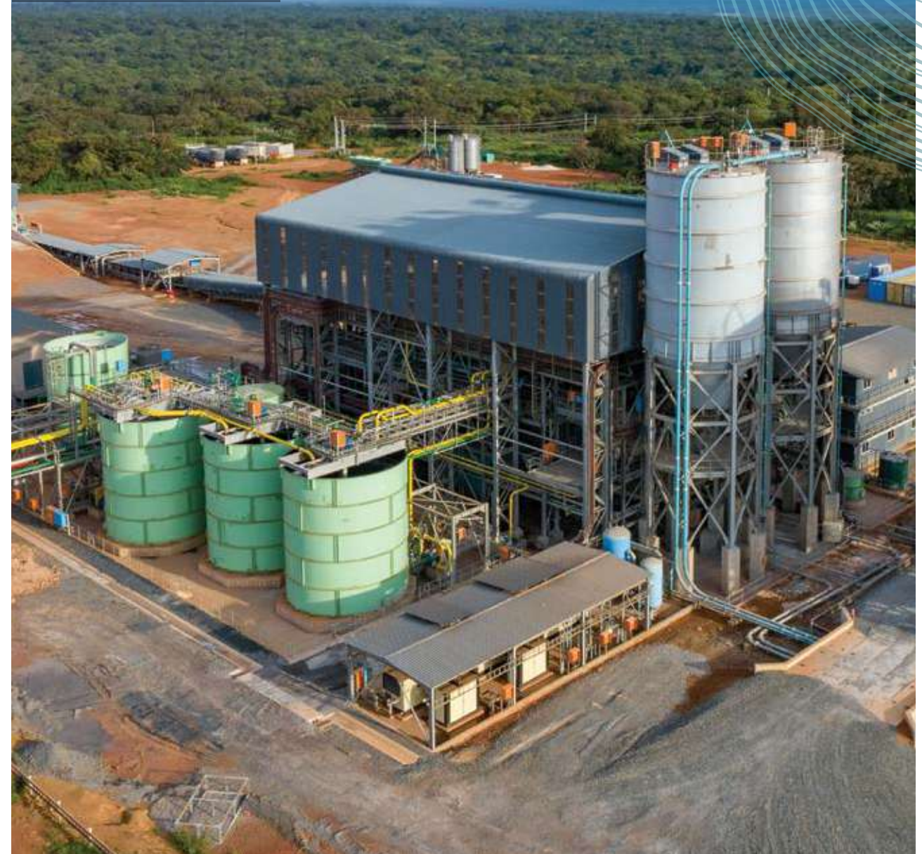
Kamoa backfill plant, South Africa
