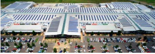
Solar farm completed at Newcastle Mall
