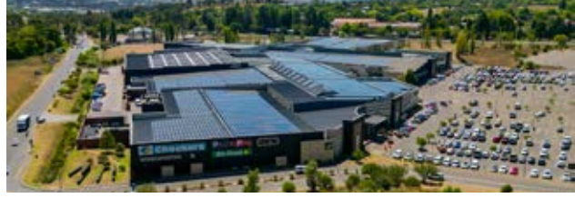
c.7 000m 2 of letting completed at Dihlabeng Mall, including 1 500m 2 new Dischem
