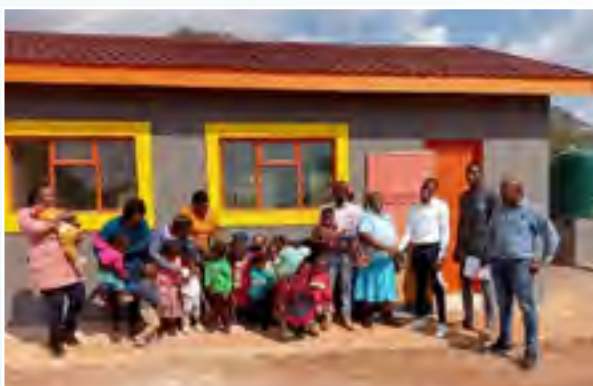
Minopex handed over a newly constructed creche in the Phalaborwa area, Limpopo, to the community.
