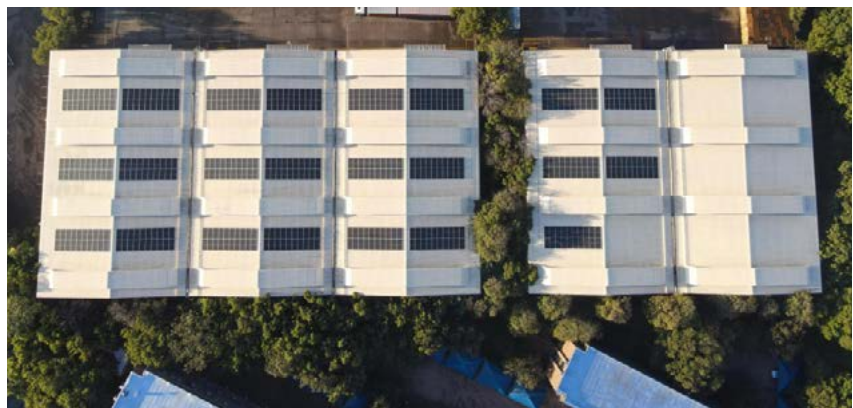
Solar installation: Builders Warehouse The Glen, Gleneagles, Gauteng GLA: 11 113 m 2
