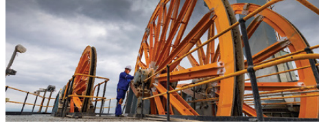
Winder upgrades increase hoisting capacity from 160ktpm to 230ktpm
